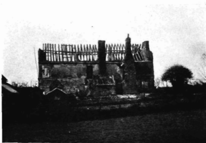
FIG. 2. HILLE'S COURT, ASH. During demolition. Back view.
